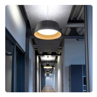
Power supply: transparent. Ceiling rose: Matching luminaire`s surface colour. High-power current. 3057lm. 32W. 4kg. Binning initial <= MacAdam 3. IP20. Protection class I. CE, UKCA marking. IK02. 220-240V. 50-60 Hz. RG0 (EN62471). Luminous flux reduction up to 0,4%/1.000 operating hours. Nominal failure rate: 0,2%/1.000 operating hours. L80B10 (tq 25°C) = 50.000h. 5 years warranty. Manufacturer: Lightnet GmbH, ISO 9001:2015 certificated.
